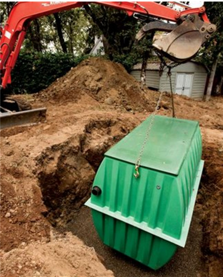
The AX-RT is a completely pre-packaged "plug & play" wastewater treatment system that can be quickly installed right behind an existing (or new) watertight septic tank.
