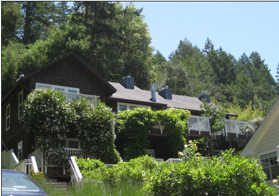
Figure 34: Inn at Occidental, 3657 Church Street. This two-story building, a modern addition to the hotel complex, stands on the hillside to the rear of the historic hotel. Its gabled roof, dark brown wood siding, and dense vegetation covering the porches, help reduce its scale and massing and make it appear to blend with the hillside.
