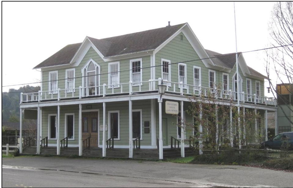
Figure 19: Hind's Hotel, 306 Bohemian Highway. Note the distinctive steeply-pitched, cross gable roof and gabled dormers.
