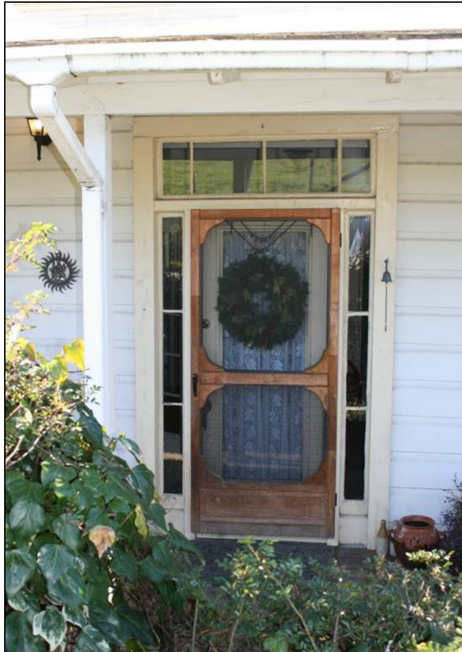
Figure 39: Screen doors and transom windows allow for natural air circulation.
