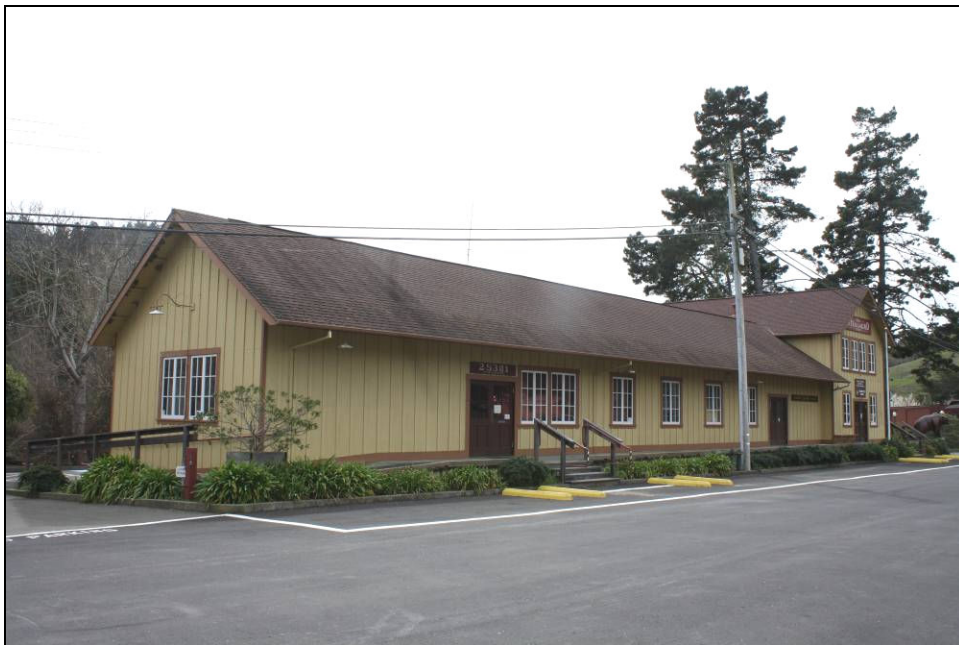
23 - 25385 Steelhead Blvd., APN 096-150-021
