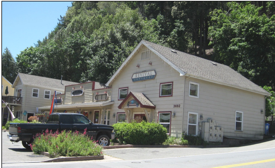
Figure 35: Commercial building, 3692 Bohemian Highway. This modern building's two-story height, front gable roof, and rectangular plan are compatible with the surrounding historic district. This commercial building maintains the existing pattern of setbacks from Bohemian Highway.
