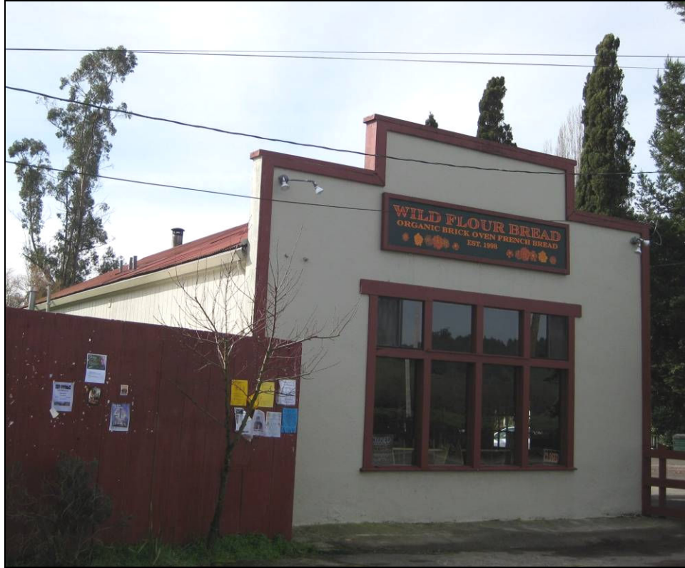
Figure 20: Commercial building, 140 Bohemian Highway. This building features a simple corrugated metal gable roof masked by a false front stepped parapet.
