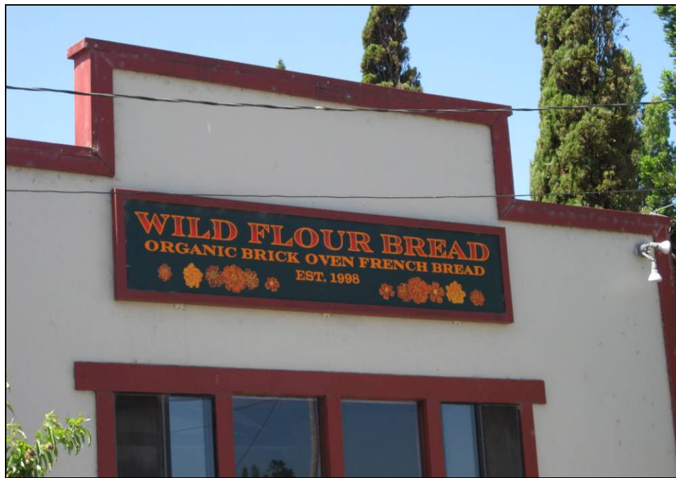
Figure 26: Commercial building, 140 Bohemian Highway. This sign on the building's façade is a good example of an appropriately scaled and designed sign. Its simple rectangular shape matches the width of the parapet and its color scheme complements the colors on the building.
