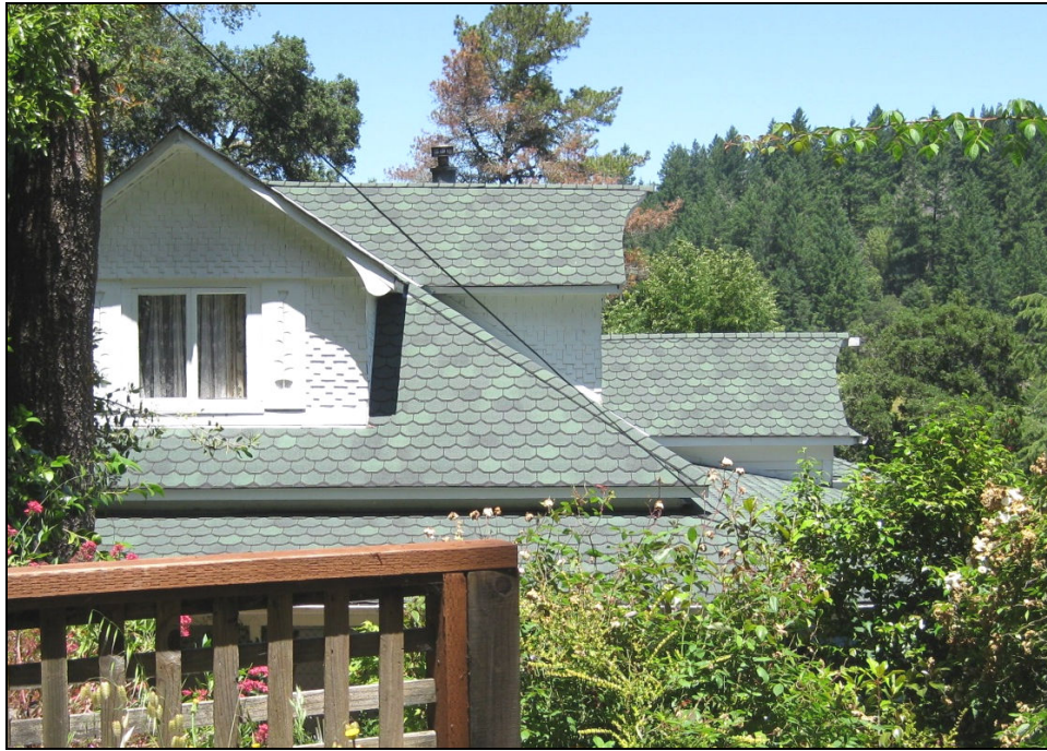
Figure 19: Residence, 14952 Coleman Valley Road. This Victorian residence features a complex roof form with prominent gabled wall dormers.
