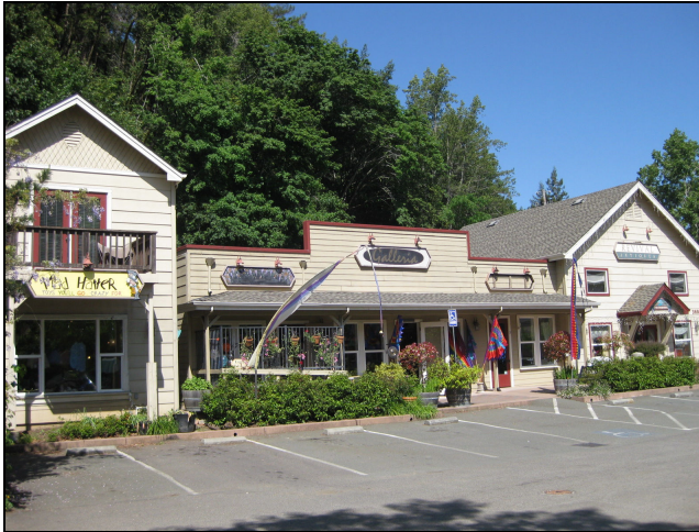
3692 Bohemian Highway, Occidental
