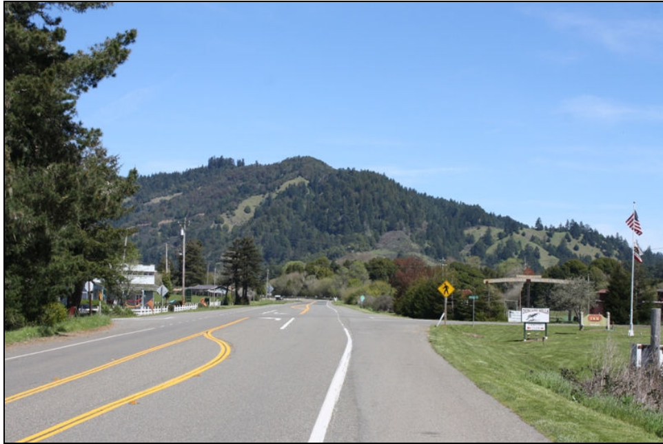
Figure 7 – View of Highway 116 with northerly shopping area to left
