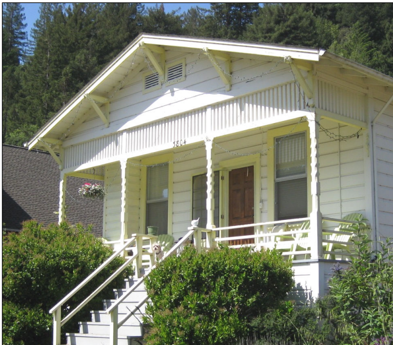
Figure 17: Residence, 3804 Bohemian Highway. This simple wood paneled door is in keeping with the style and character of this vernacular circa 1880 cottage
