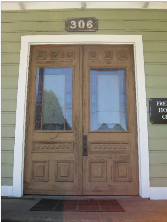
Figure 18: Hind's Hotel, 306 Bohemian Highway. Although they may not be the building's original doors, these paneled, glazed wood double-leaf doors are in keeping with the style of the building and original openings have been retained.
