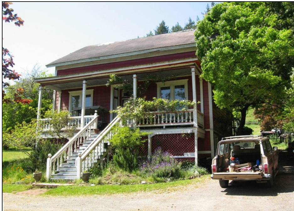
Figure 16 - Porch on the historic Supervisor's Building
