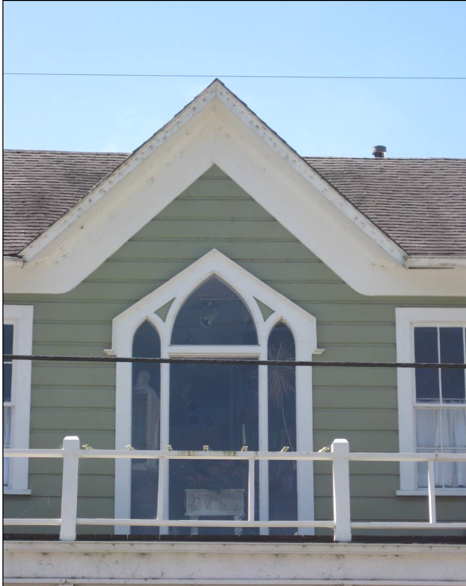
Figure 17: Hind's Hotel, 306 Bohemian Highway. The distinctive Gothic arched windows on the second story are an important character-defining feature of the building and should be preserved.
