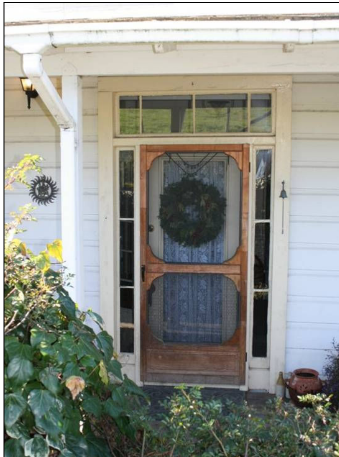
Figure 38: Screen doors and transom windows allow for natural air circulation
