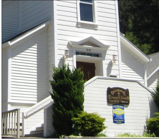
Figure 18: Occidental Community Church, 3637 Church Street. The door's centered location on the façade and prominent gabled pediment and transom are important character-defining features that should be preserved.
