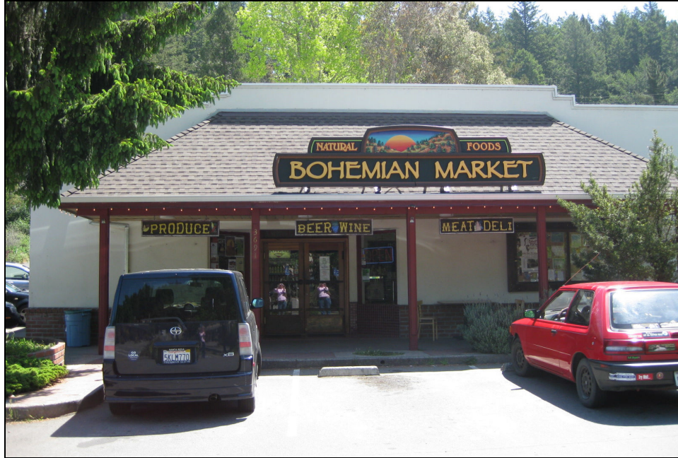
Figure 27: Commercial building, 3633 Bohemian Highway. The signage on this commercial building is compatible with the character of the surrounding historic district. The primary sign on the porch roof is well designed and scaled to the building. The signs clearly communicate the name of the business, while secondary small hanging signs advertise specific items for sale.
