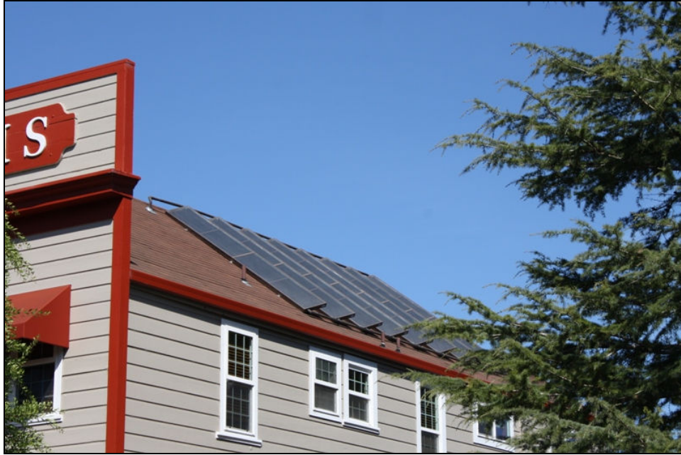
Figure 38: Solar panels discretely placed on a side gable behind the false front.
