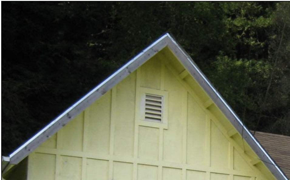
Figure 13: Residence, 460 Bohemian Highway. This addition has new board-and-batten siding that is compatible with the neighborhood.
