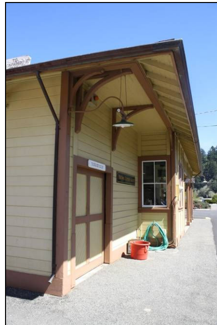
Figure 23 - Gooseneck light on train depot
