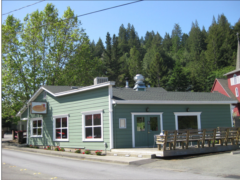
Figure 36: Commercial building, 3782 Bohemian Highway. This building's one-story height, wood siding, and simple fenestration complement the surrounding historic district. Similar to other historic buildings located across the street, this building has a minimal setback from the street
