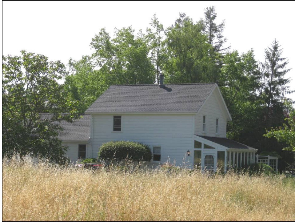
Figure 32: Residence, 425 Bohemian Highway. The gabled addition is located on the rear elevation of the historic home. The addition's one-story height is subordinate in size to the historic house while its roof form and siding are also compatible and in keeping with the style and character of the historic house.
