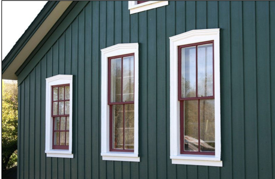
Figure 11 - Double-hung windows in Bodega Historic District
