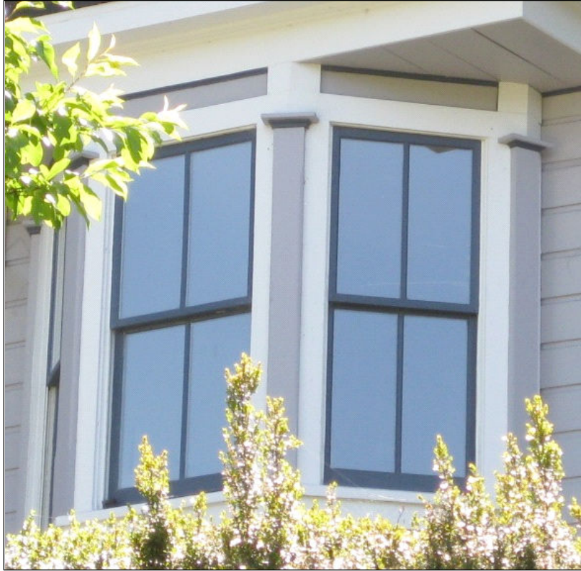
Figure 15: Residence, 14895 Coleman Valley Road. Although the original windows may have been replaced, these two-over-two, double-hung windows maintain the original windows' historic configuration, operation, details and finish and the distinctive window surrounds have been maintained.
