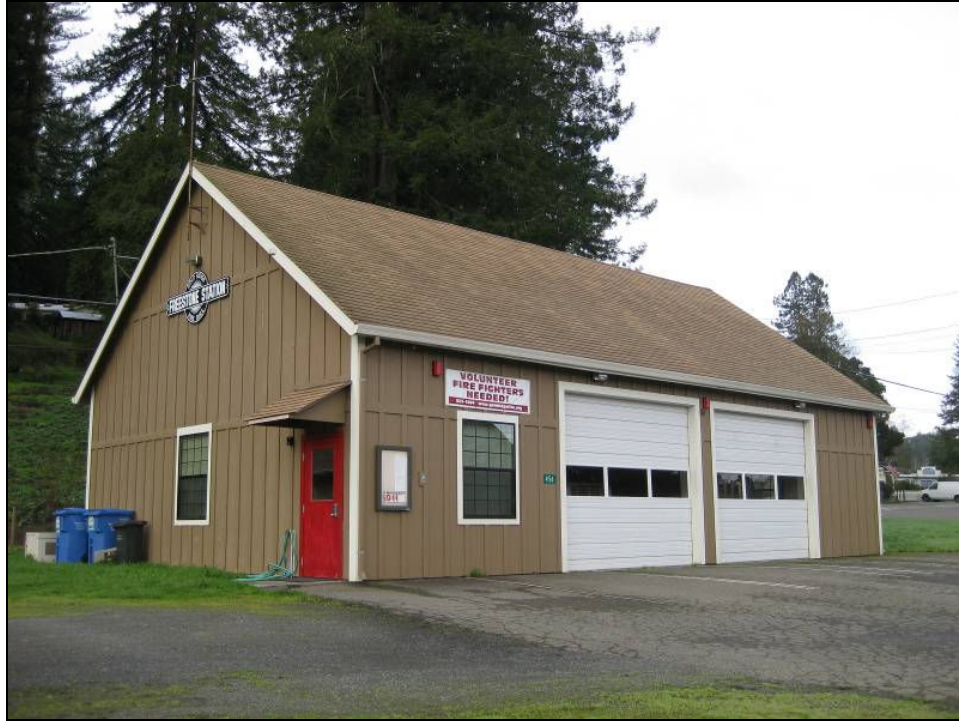
Figure 33: Gold Ridge Fire District's Freestone Fire Station, 456 Bohemian Highway. The building's one-story height, steeply-pitched gable roof, and board-and-batten siding are compatible with the surrounding historic district. The building's orientation parallel to the street is a common characteristic of surrounding buildings in the historic district.
