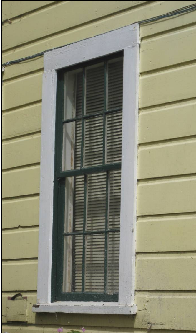
Figure 16: Commercial building, 500 Bohemian Highway. This building retains some original, wood six-over-six, double-hung windows with simple surrounds.
