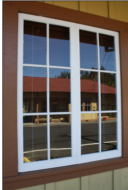
Figure 13 - Casement window in Duncans Mills
