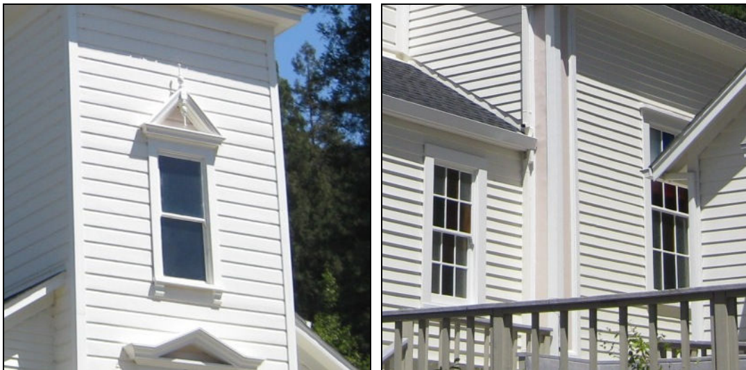
Figure 16: Occidental Community Church, 3637 Church Street. The distinctive central window on the front façade featuring a pediment surround (left) and the wood, six-over-six, double-hung windows (right) are character-defining features of this building.
