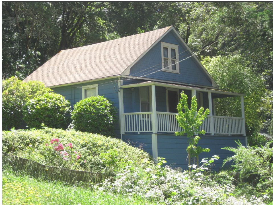
Figure 20: Residence, 14717 2nd Street. This building features a simple front gable roof.
