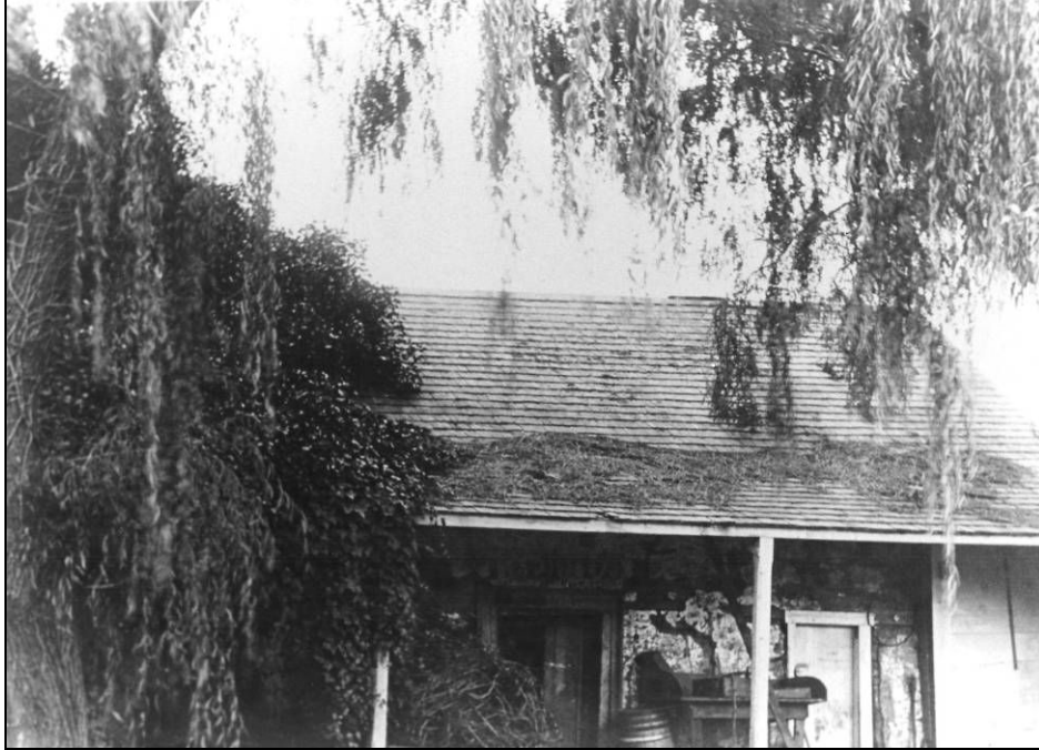
Figure 1: The O'Farrell adobe house on Analy Ranch owned by Jasper O'Farrell in Freestone (Courtesy of the West County Historical Society, Sebastopol). This building was built by James Black prior to 1844.
