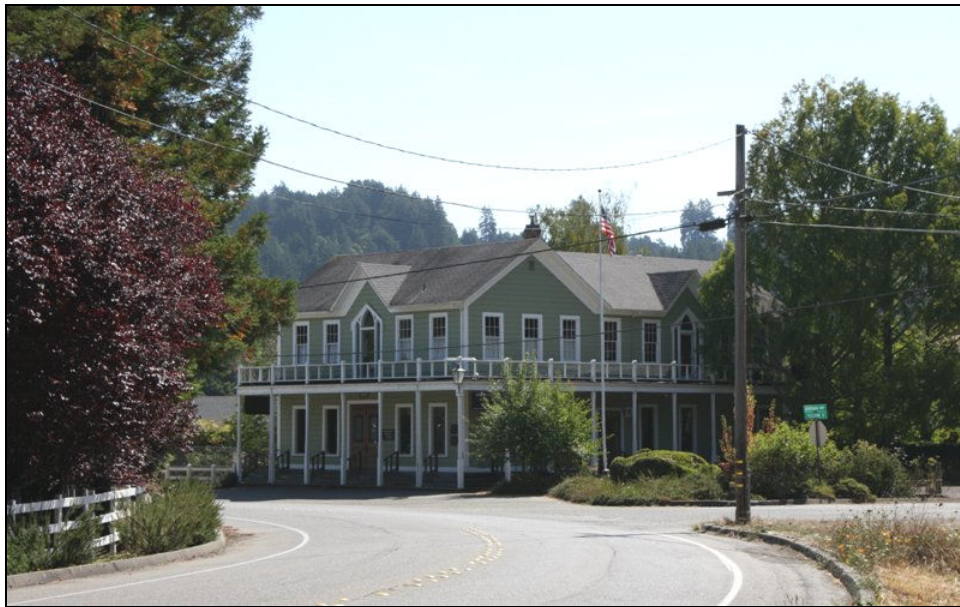
Figure 9 - View of Freestone House from the north, traveling on Bohemian Highway
