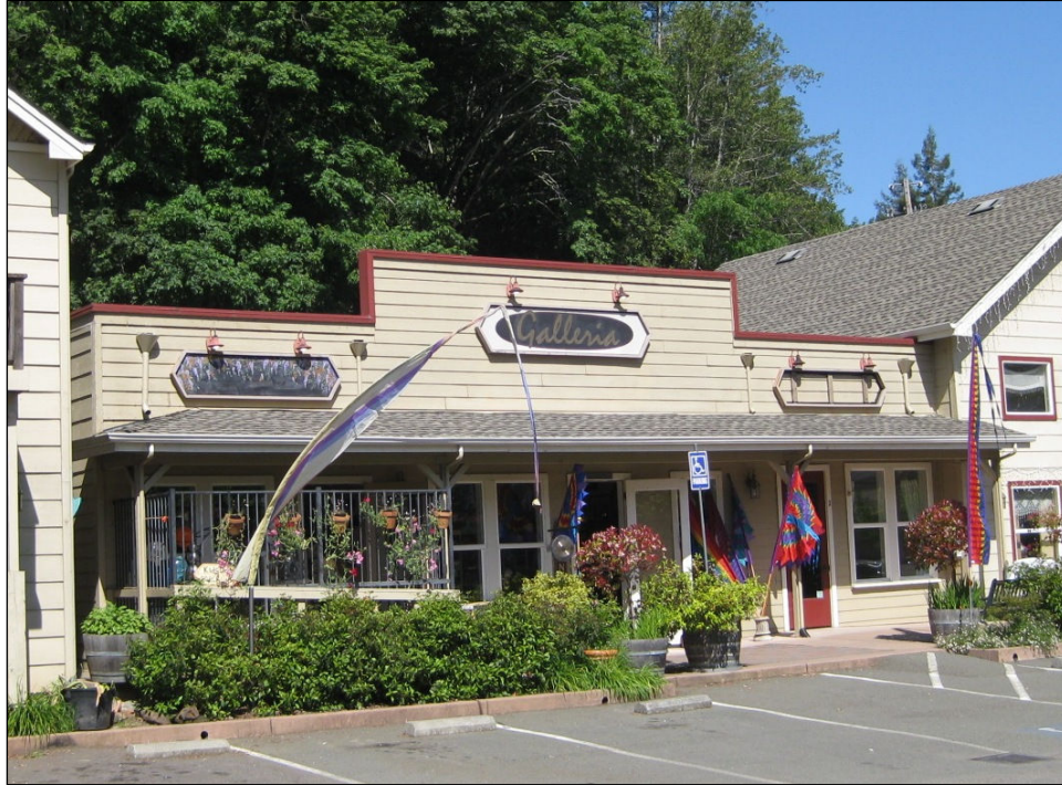
Figure 25: Union Hotel, 3731 Main Street. The full-width wood awning that wraps around the side elevation provides scale, character, and shade on this commercial building. Its wood construction is typical of awnings located on buildings within this historic district.
