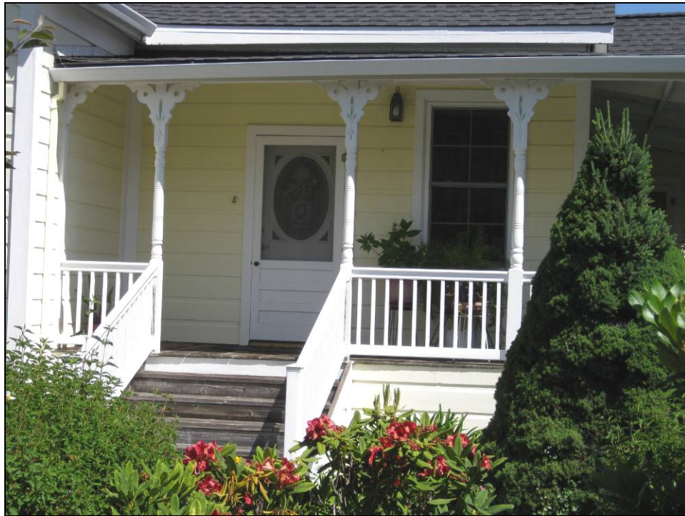
Figure 21: Residence, 301 Bohemian Highway. Although the bracketed porch supports and open railing are likely not original, the details of the porch are in keeping with the style and scale of the building. In particular, the height of the railing and spacing of the balusters are appropriate for the porch.
