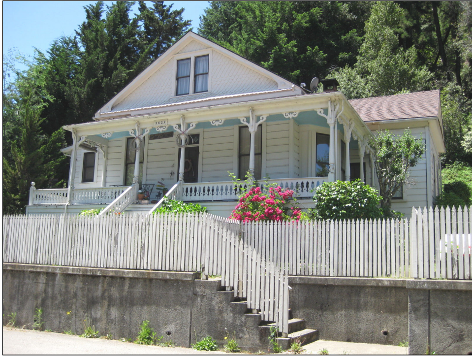
Figure 23: Residence, 3622 Bohemian Highway. This building appears to have retained its original porch, including its turned posts, scrolled brackets, and distinctive balustrade. These important character-defining features should be preserved.
