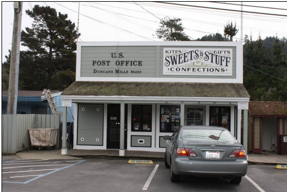
23 – 25375 Steelhead Blvd., APN 096-150-021
