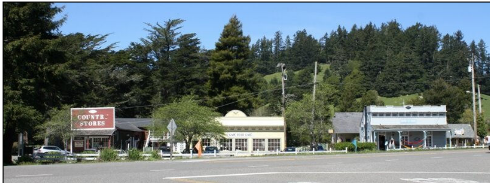
Figure 8 - Northerly shopping area looking west
