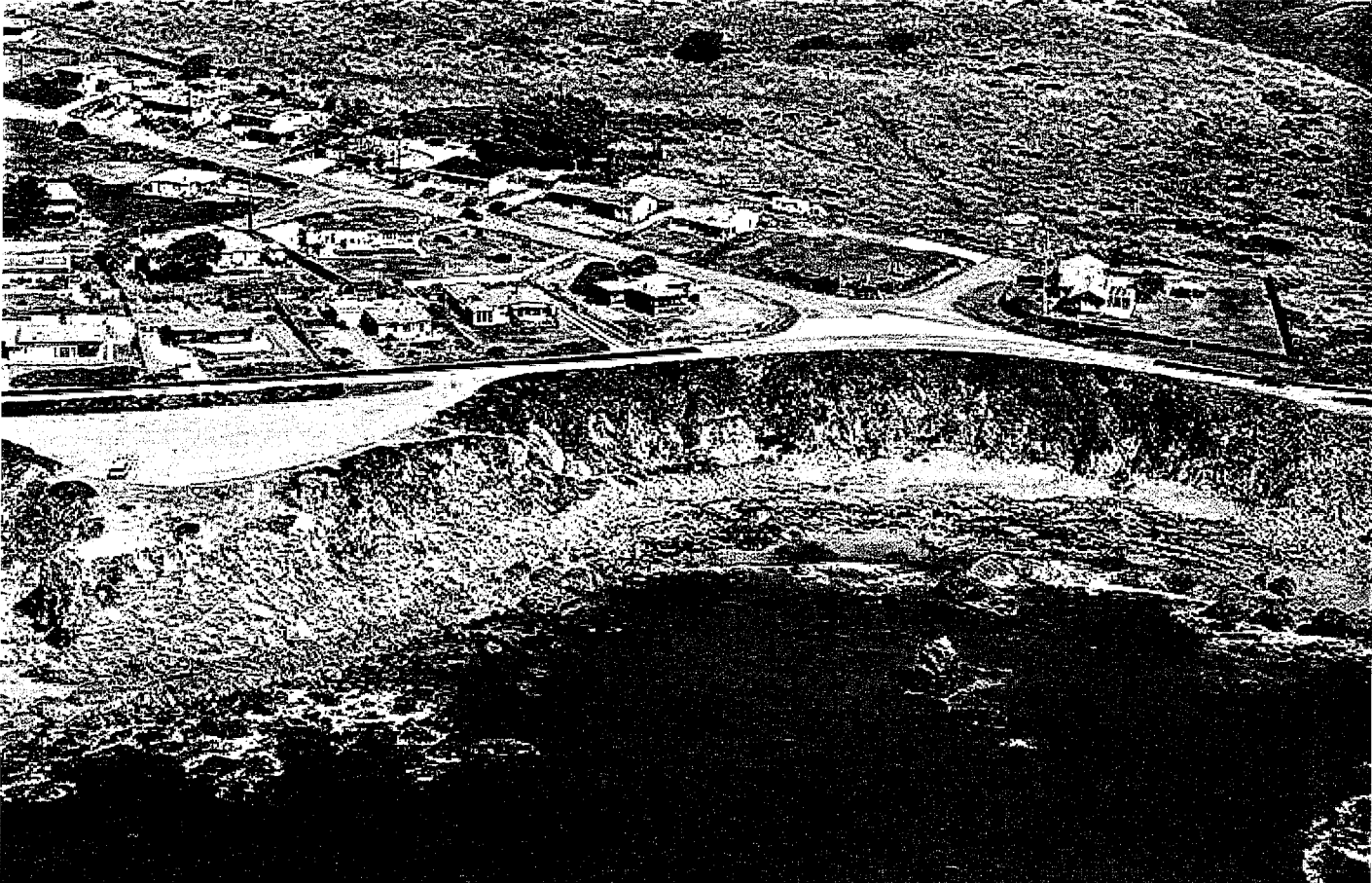
Highway 1 near Carmet Drive – across from Carmet Beach access
