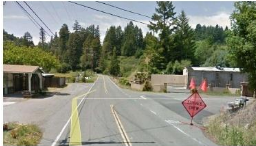
Hwy 116 near Odd Fellows Park (looking westerly)
