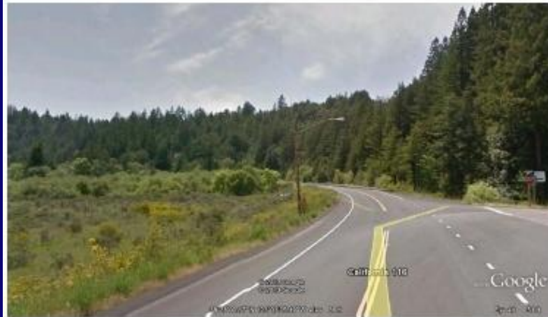
Hwy 116 at Cazadero Road (looking westerly)
