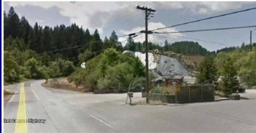
Hwy 116 near Giovanetti Rd (looking westerly)
