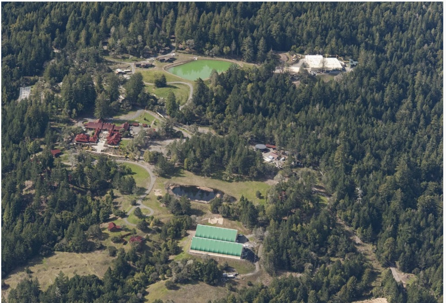
An aerial view of the Ratna Ling Retreat Center. Photo: Coastal Hills Rural Preservation
