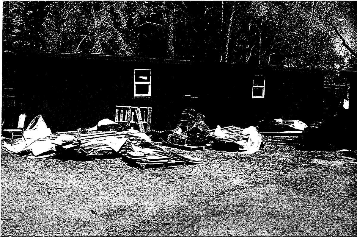
Figure 6. Existing storage building.
