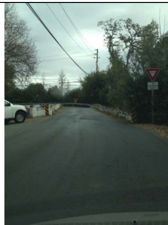
Laughlin Bridge Northerly Approach
