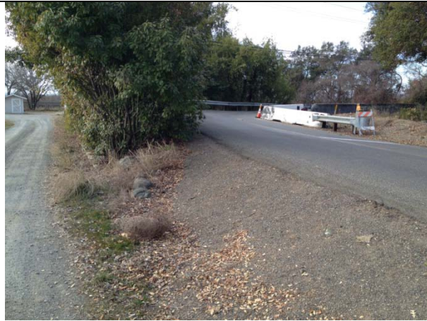
Laughlin Bridge Southerly Approach
