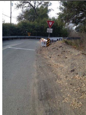
Laughlin Bridge Southerly Approach
