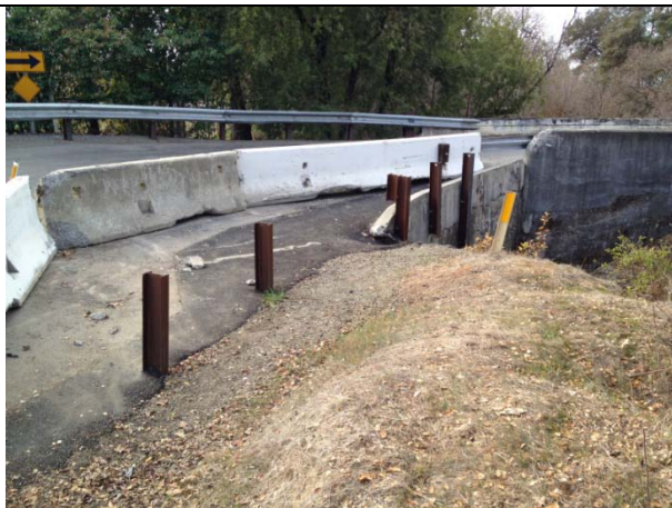
Laughlin Bridge Southerly Abutment
