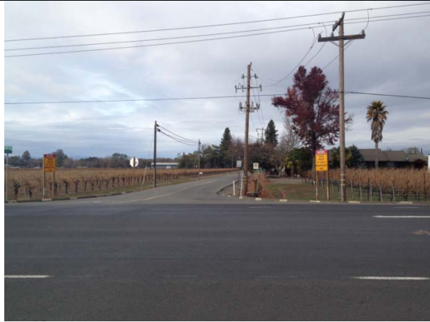
Advanced Warning Signage River Road @ Laughlin Road
