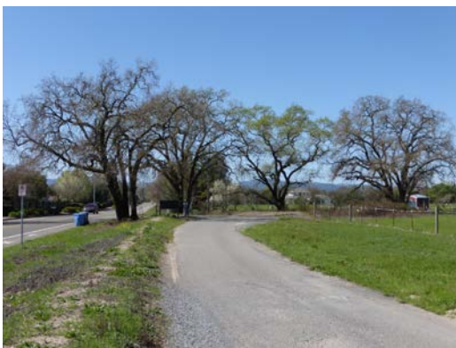
Figure 1. View of proposed road from Arata Lane to the left (looking west)
