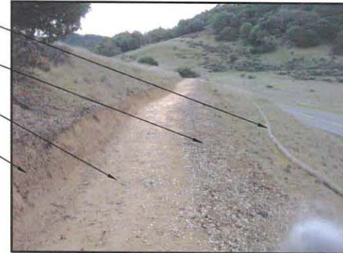
NEW FULL BENCH CONSTRUCTION- COMPACTED SOIL TREAD
