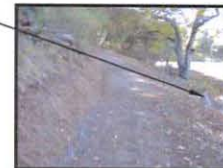
NEW FULL BENCH CONSTRUCTION- STABILIZED AGGREGATE TREAD
