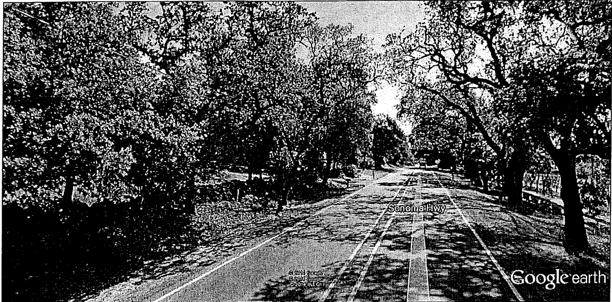
Figure 18: Subarea 2 - street view between Cavedale and Moon Mountain
