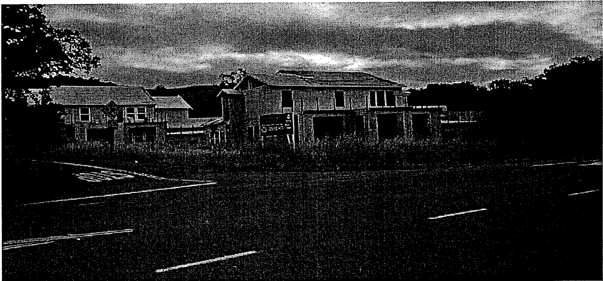
Figure 26: Subarea 3 - photo May 2014 of 6 bedroom house/second dwelling unit/garage under construction
