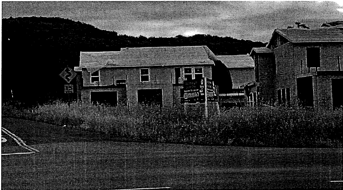
Figure 24: Subarea 3 - photo May 2014 of 6 bedroom house/second dwelling unit/garage under construction
